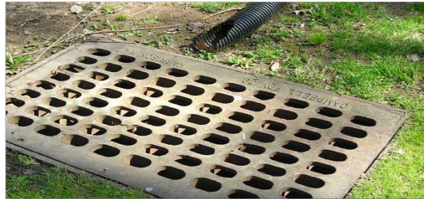
Drainage grate in back yard
