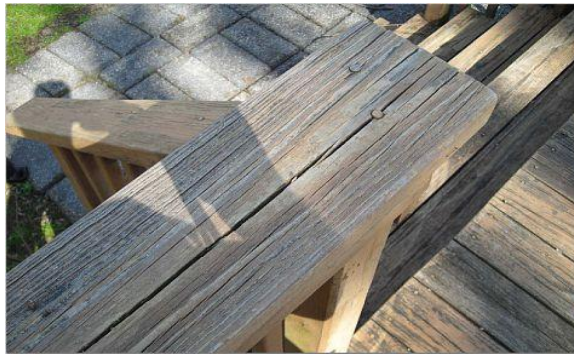
Splitting railing top board
