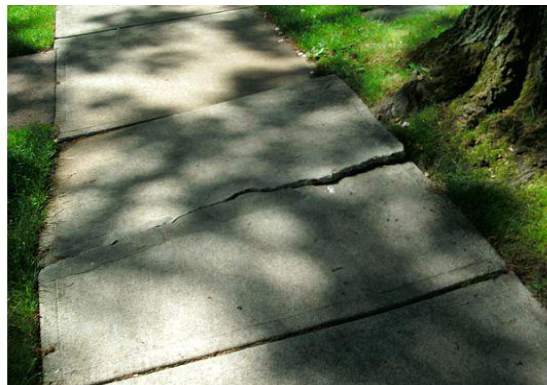
Cracked sidewalk
